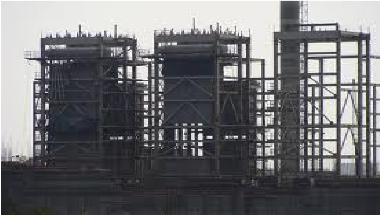
Waste to Energy Plant, Timarpur
